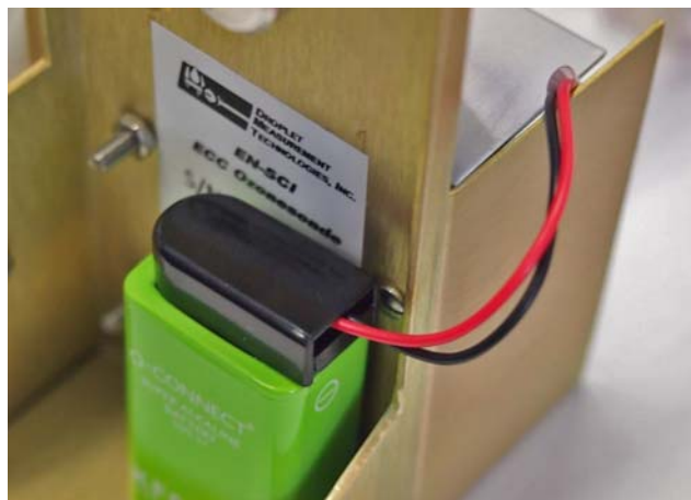
Figure 33 Battery Wires Running Between the Ozone Sensor Frame Wall and the Ozone Sensor
